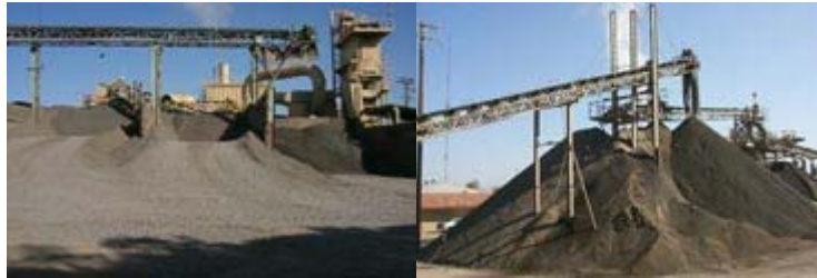
Stockpile and Conveyor System
